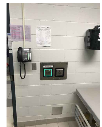
WASHROOM SIDE W/OUTWARD SWINGING DOOR "PUSH TO OPEN" AND "PUSH TO LOCK"
